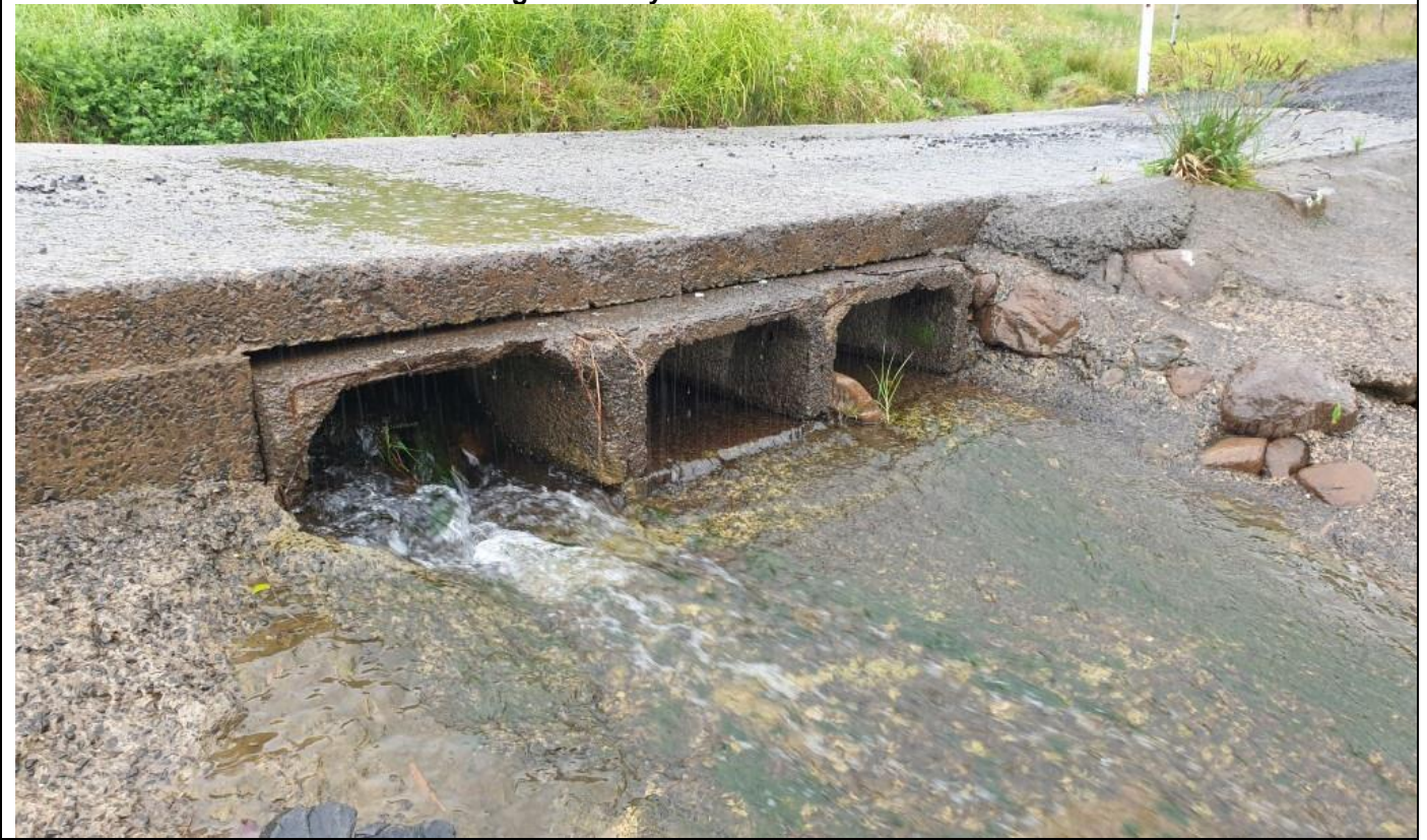
Photo 11. Box culverts beneath existing causeway
