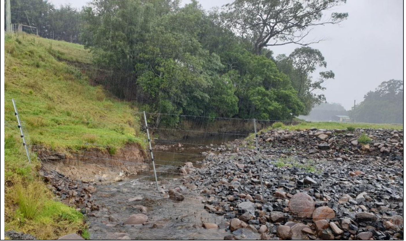
Photo 9. East of causeway –in-stream cobbles to be removed and used in Kyowa bags for scour protection
