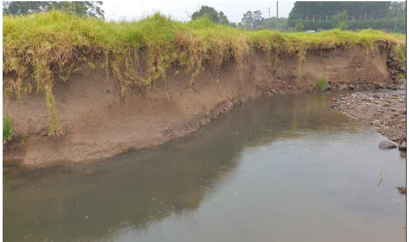
Photo 8. Eroded clayey scarp to the west of Martinvale Lane – scour protection proposed and deep pool to be filled
